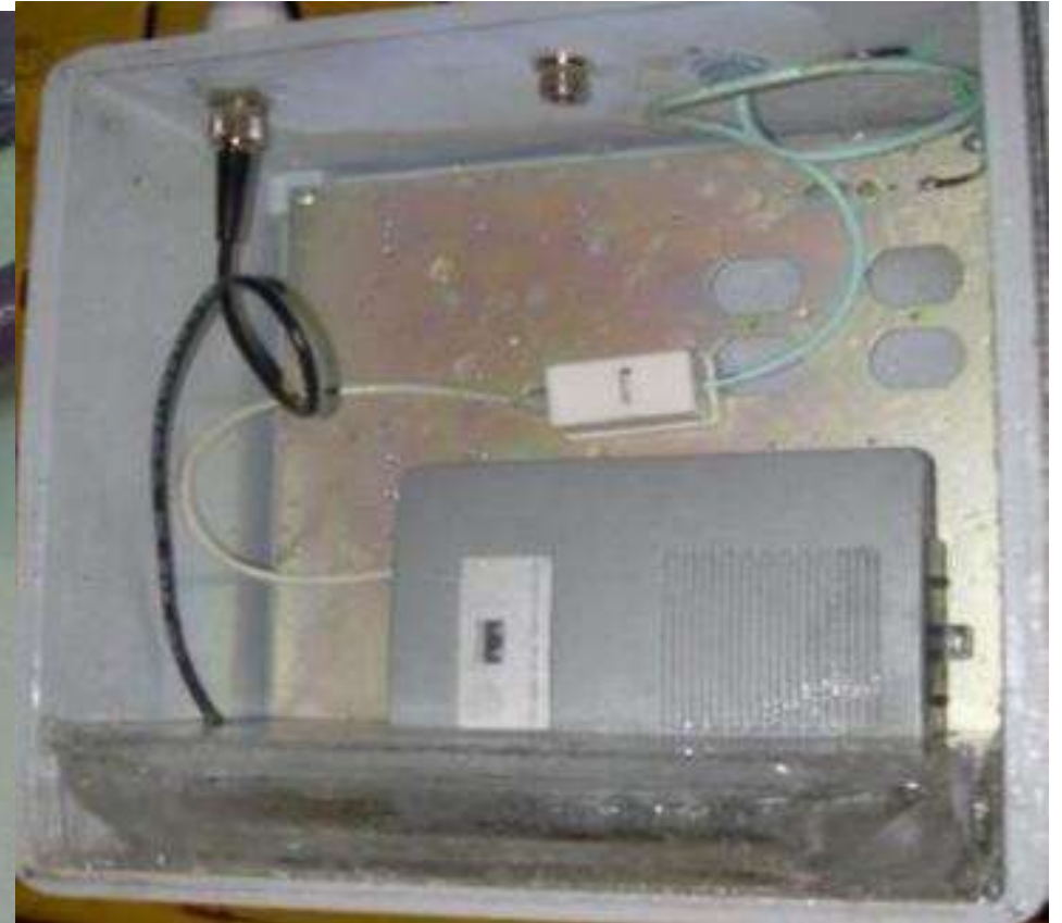
Outdoor NEMA box not weatherized (just keeping the packets on ice)
